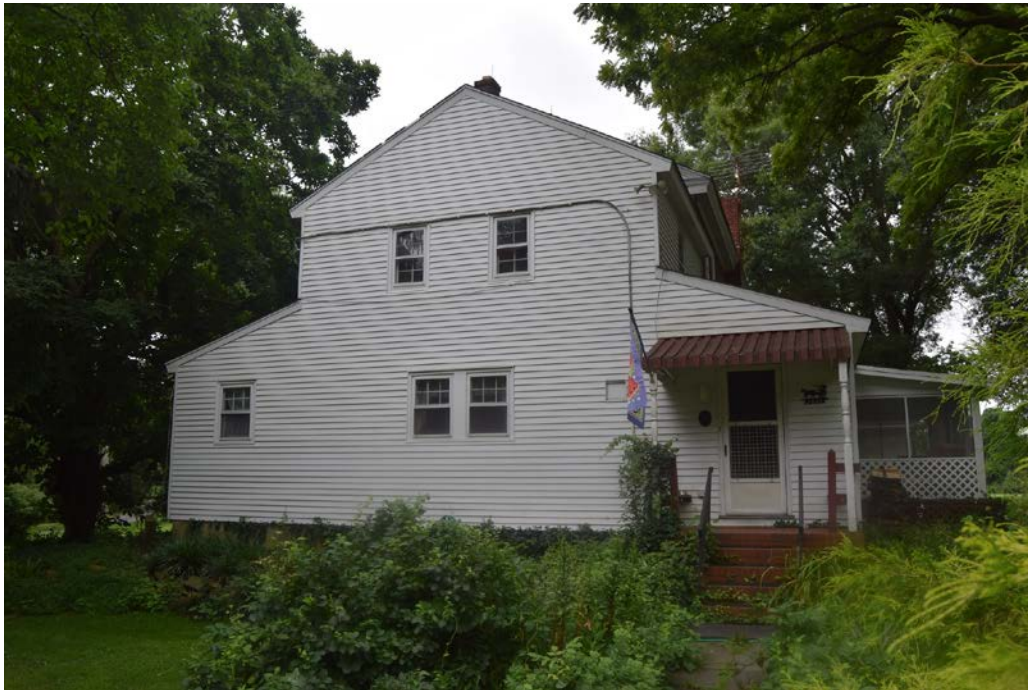
Photo 9. Northeast side of house toward southwest.
